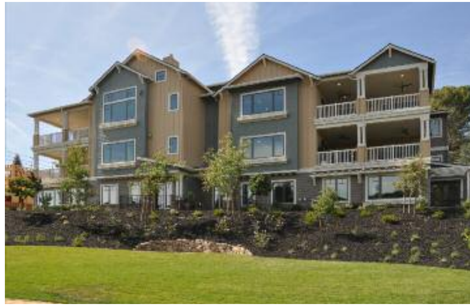
The first of six Woodbury luxury condominiums in Lafayette.
